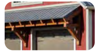
Open Rafter Awning
