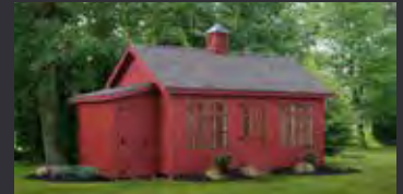
Shed Addition page 42
